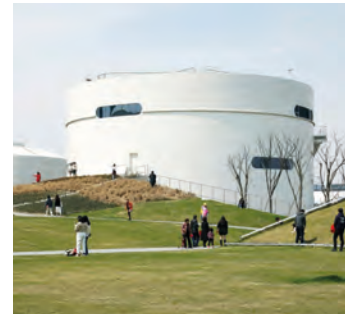
Abb. 168: Transformation Silo zu Museum
